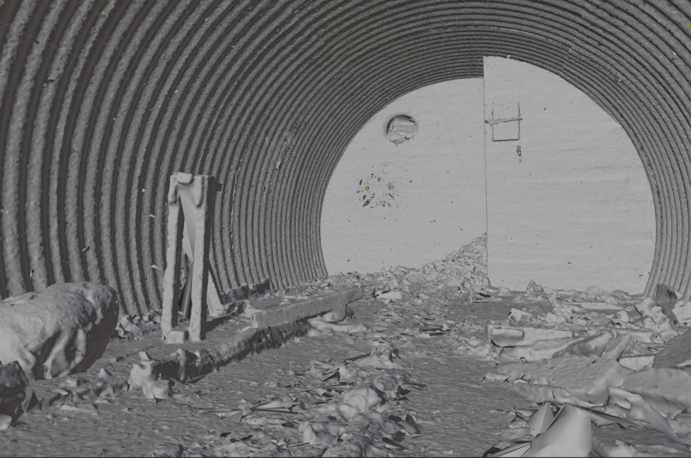
3D view of the bunker interior based on solid mesh data.
