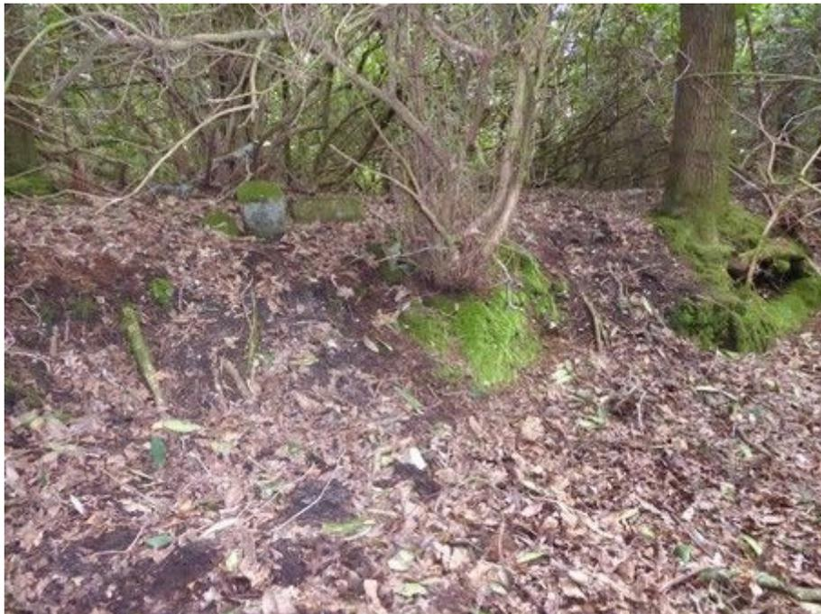
Photo 2: View from within the main chamber area. To the left of the central tree are loose hollow concrete blocks. To the right can be seen the curved tops of two glazed earthenware pipes that formed part of the ventilation system.
