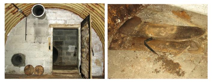
The floor of the radio room was originally covered with a layer of brown linoleum, small sections are still in place (above right) and some of these bear indents of objects that stood on them. Three aerial feeder cables emerge at about 40 cm above floor level near the right-hand corner, near the entrance doorway (below left). The presence of three feeder cables indicates that three aerials – each one on its own tree – were used. The table for the radio sets would have stood near this corner.
