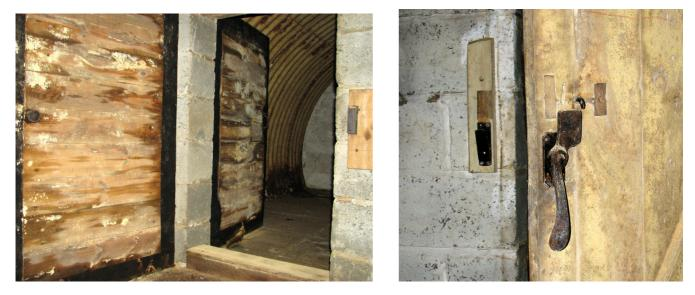
The two aforementioned concrete ventilation pipes traversing the generator room emerge in the radio room, to the left of the twin doors (viewed from the entrance doorway). Their homemade plugs (used for noise reduction) are in situ. In the radio room
