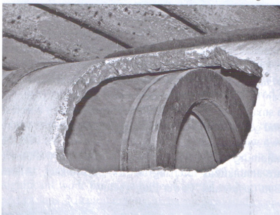
Outlet ventilation pipe with extractor fan mounting
