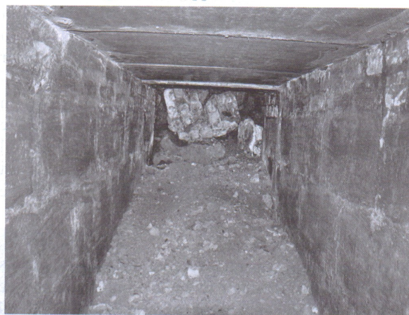
Emergency exit tunnel
