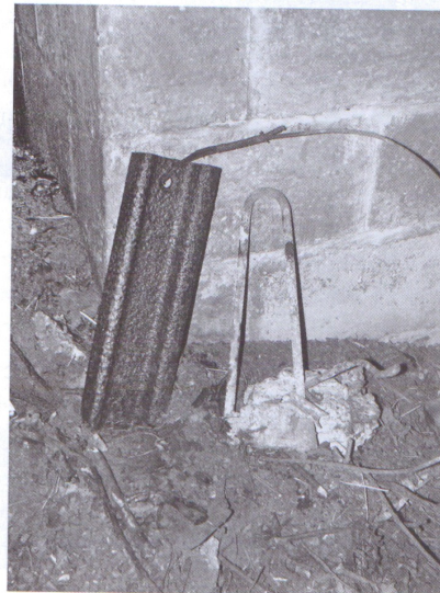
The counterweight – a length of 95 lb bullhead railway
