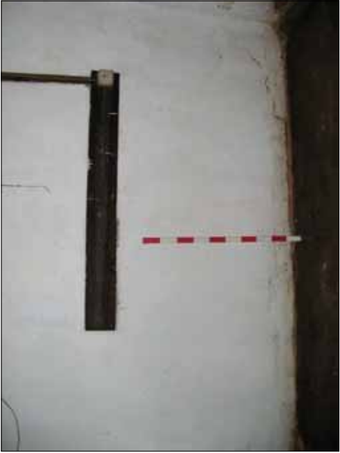
Plate 13: Bunker switch board
