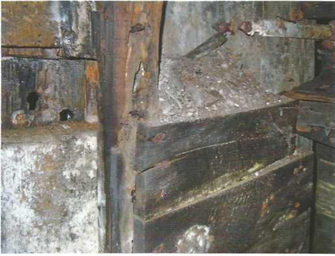
Inside view of the blast door
