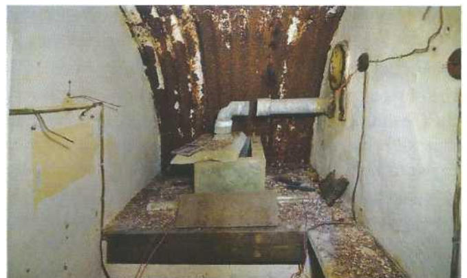
Exhaust box for generators. Photo Chris Warren
