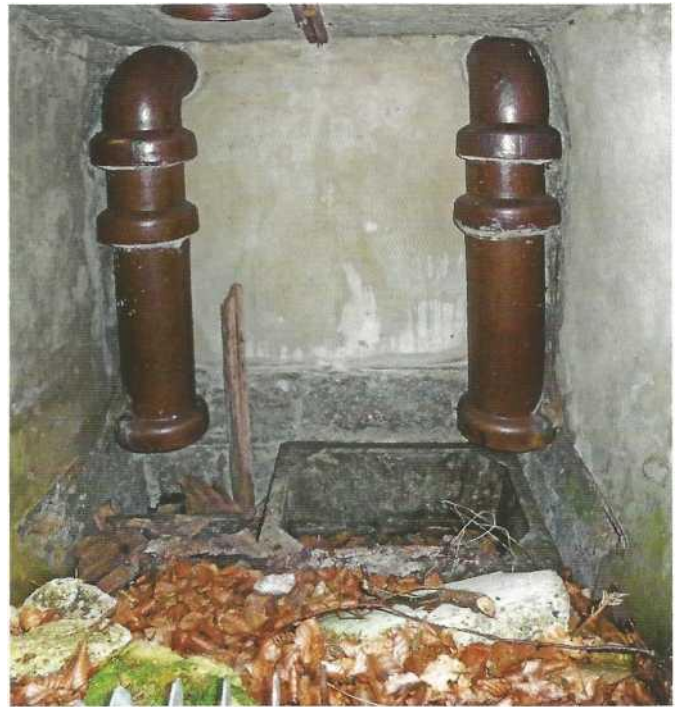
Ventilation pipes near tunnel exit
