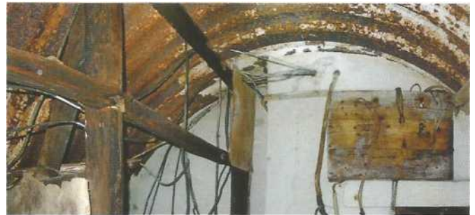
Cable Distribution Panel
