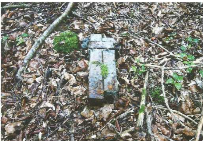
Counterweight for hatch
