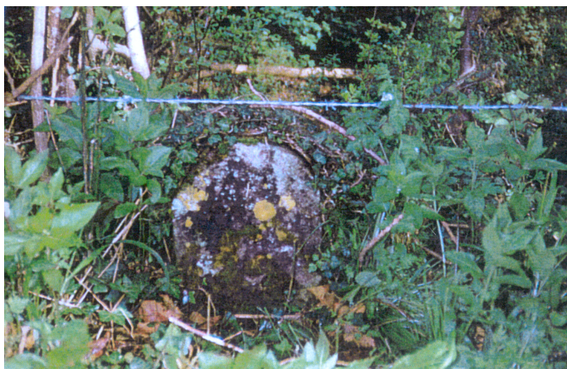
Escape tunnel exit.
