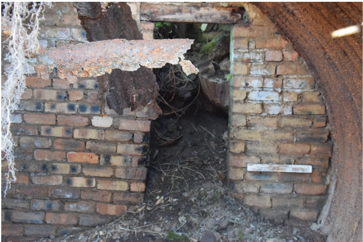
Image © David Blair. Door aperture that leads into the curved double walled escape route, right turn
