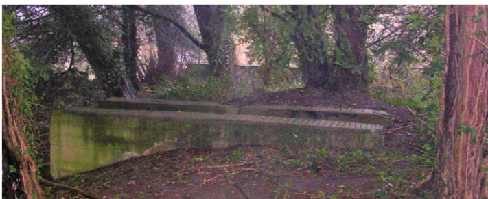
The Inspection Service Ramp
